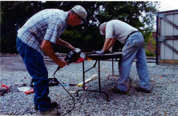
Bob Hooper assists Glenn Terminelli of the Phillipsburg Railroad Historians in preparing a vital brake system link for welding to increase its length. Tony Hall photo, 6 August 2011.
