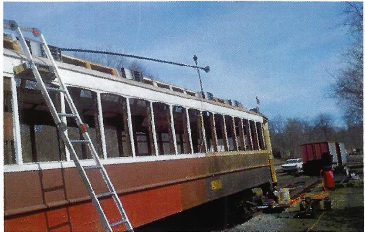
Poles crossed in the temporary absence of pole hooks in preparation for safe ingress into carbarn. Photo Tony Hall, 10 Mar 2012.
