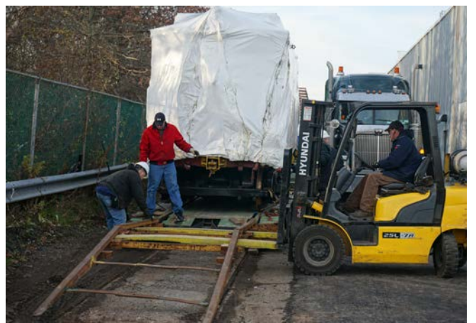
Figure 18: The unloading ramp is once again deployed.
