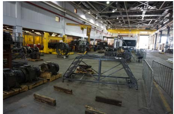
The vastness of the NJT's HBLR maintenance facility is seen in this view. This space is required when you have a strong maintenance program.
