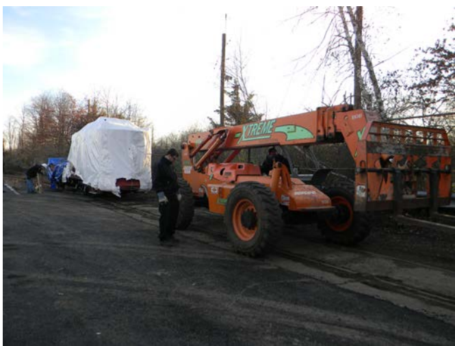
Figure 15: KS Fork Lift pulls Flat Car 5223 from its temporary overnight storage location.
