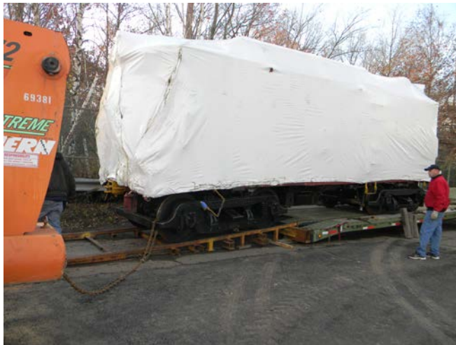
Figure 21: Gravity gets some help as the forklift pulls the car and the cable slowly plays out from the winch.
