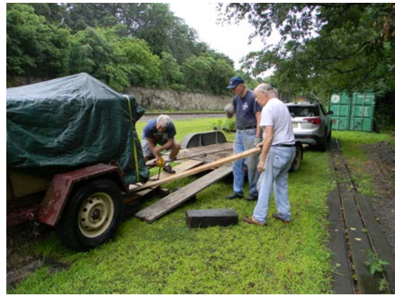
Ken Miller's trailer is coupled to Bob Hooper's vehicle as Bob, Hank and Ken assemble the loading ramp.
