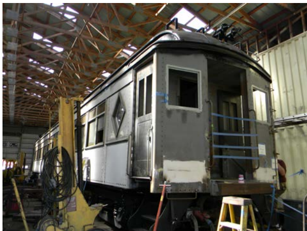
After a long campaign, the Whippany Railroad Museum's Lackawanna Parlor car approaches completion.
