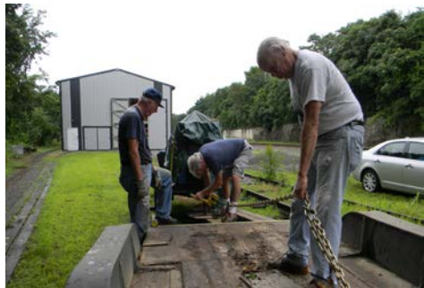
Rigging a come-along, our intrepid trio prepares to tow the generator up the ramp onto the trailer.
