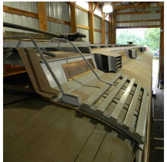
Clerestory glass, ventilators and trolley poles were recently joined by the application of the roof access ladders.
