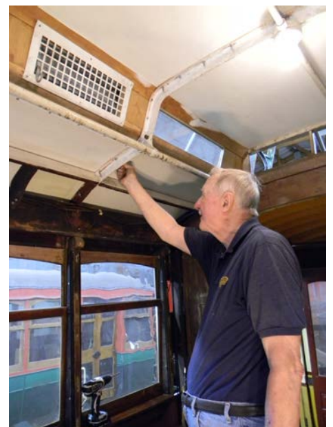
Hank tightens the last of the roof access ladders bolts.
