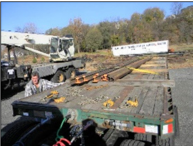
Fig. 8-6. Ten lengths: loaded, secured and ready to roll! DSCN4003
