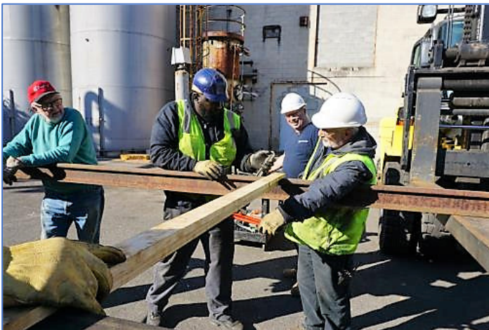
Fig. 9-5. The gauge is checked and re-checked before the panel is placed.
