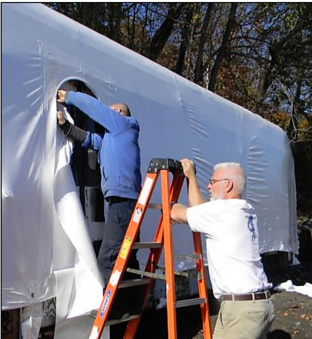
Fig. 7-5. ACCESS PORT ADDED. DSCN3924
