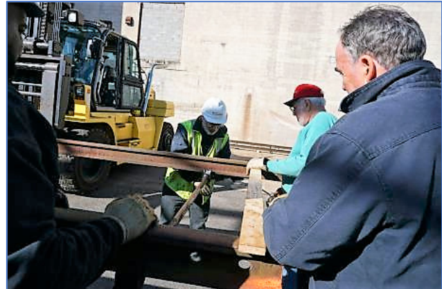
Fig. 9-4. Track panels are assembled as Bob Hooper, Captain Bill and Mike Healy supervise. DSCN6144
