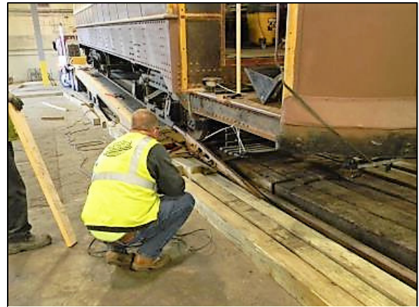
Fig. 18-4. With precise alignment finally achieved, unloading can begin.
