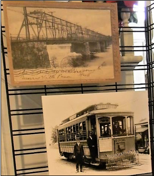
Fig. 6-1. Trolley bridge over Delaware River and a car in service. DSCN4271
