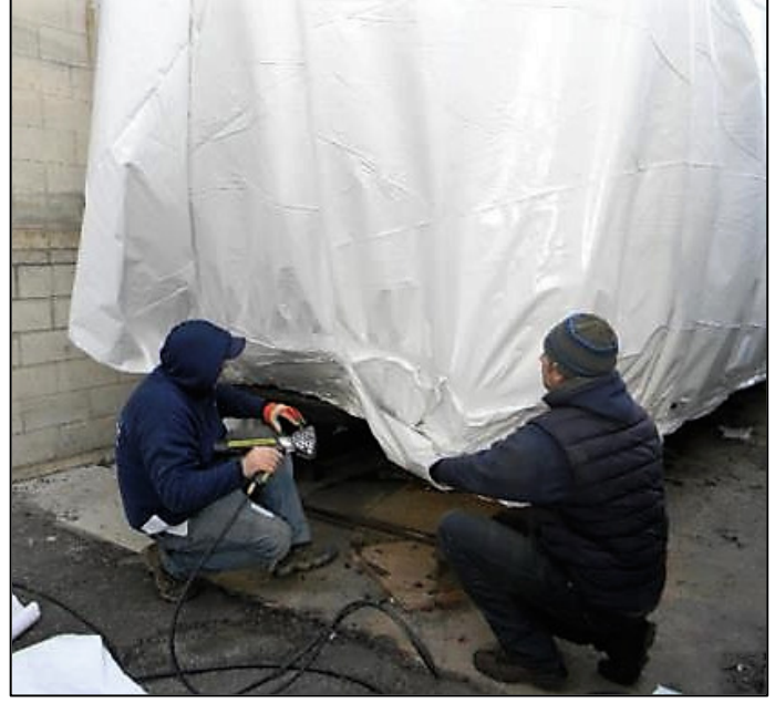
Fig. 14-1,2. Welcomed heat is applied to shrink the wrap.
