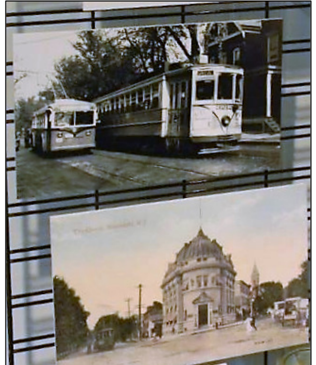
Fig. 6-2. Equipment in service and view of Bloomfield Avenue at Broad Street in Bloomfield. DSCN 4272
