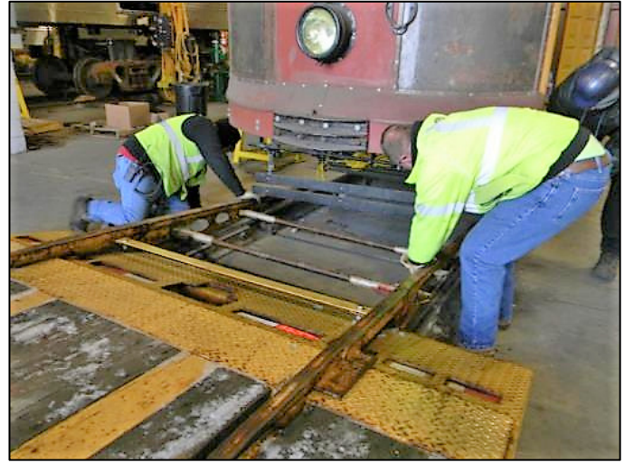
Fig. 15-2. The ramp is assembled.
