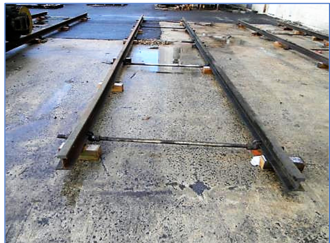
Fig. 9-6. Three track panels are ready to receive our cars.
