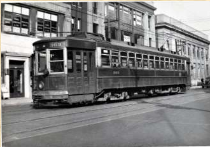
Fig. 6.5 Passing the now unobstructed entrance to a handsome Art Deco office building, Car 363 glides unfettered to her destination. This location was a hot spot for 1930's trolley photographers. Thank Goodness! (Keigher Collection p151l)
