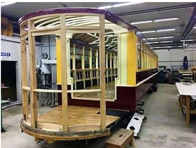
Fig. 14.3 End platforms have taken shape. (IN-7)
