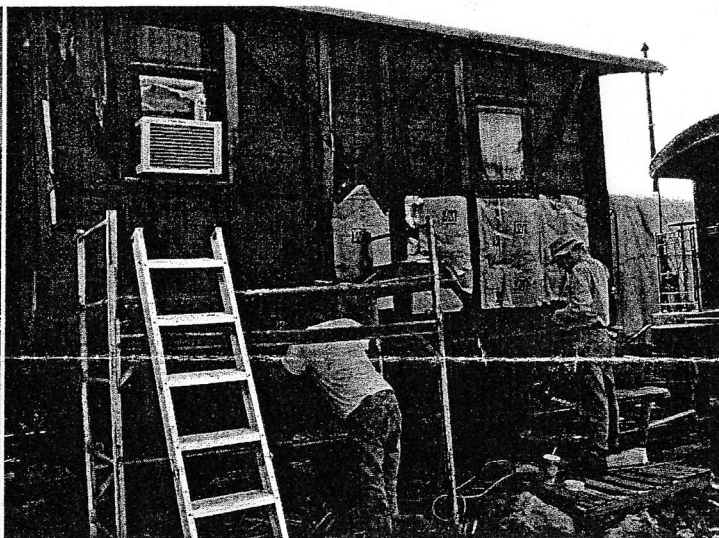
Denny Pacelli and Gene Carson have removed the old rotted sheathing from LNE 516. Note the typical wooden construction. The window on the right was later blanked to simplify this re-sheathing. (R. Slinsky)
